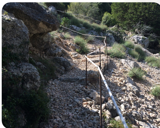
Trail conditioning with a low mesh of galvanised triple torsion steel, laid on the rocky bottom and anchored with galvanised steel wire. In the image on the left, we can see mules carrying fencing material. Yew grove of Cosp (Cardó Mountain). Photos: Jordi Bas and Jordi Camprodon.
