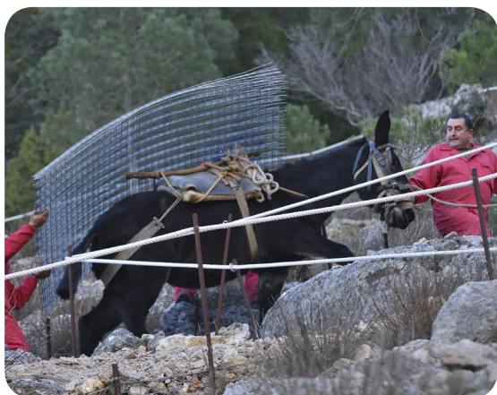
Trail conditioning with a low mesh of galvanised triple torsion steel, laid on the rocky bottom and anchored with galvanised steel wire. In the image on the left, we can see mules carrying fencing material. Yew grove of Cosp (Cardó Mountain). Photos: Jordi Bas and Jordi Camprodon.
