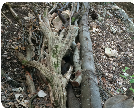
Faggot revetments to prevent erosion in the mature yew forest of Cosp (Cardó Mountain). Branches and twigs from competition regulation works were reused. Photo: Jordi Camprodon.
